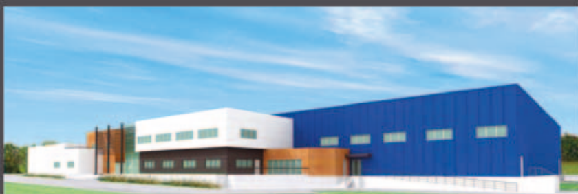
New offices with High Quality Environmental standards
